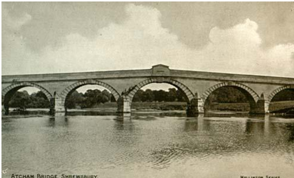
Atcham Bridge (ref: PC/A/27).
