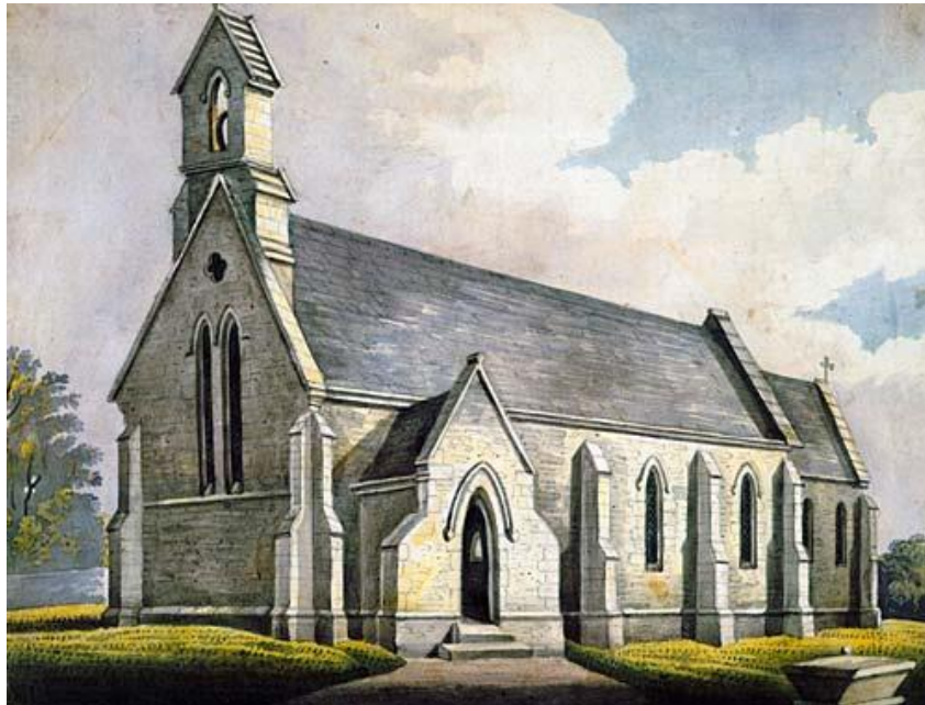
St Mary's Church, Eaton Constantine rebuilt during the 1840s on the site of a much earlier church
