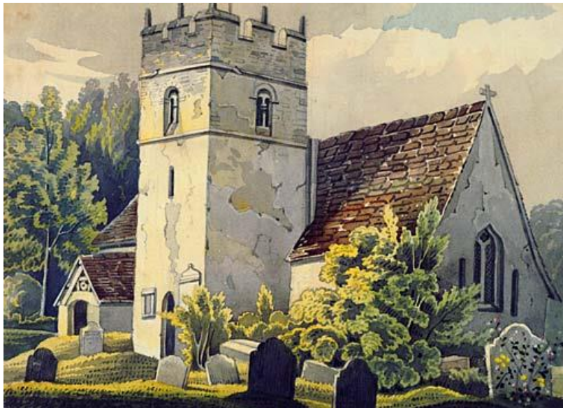
St Edith's church, Eaton-under-Heywood before restoration in 1868
