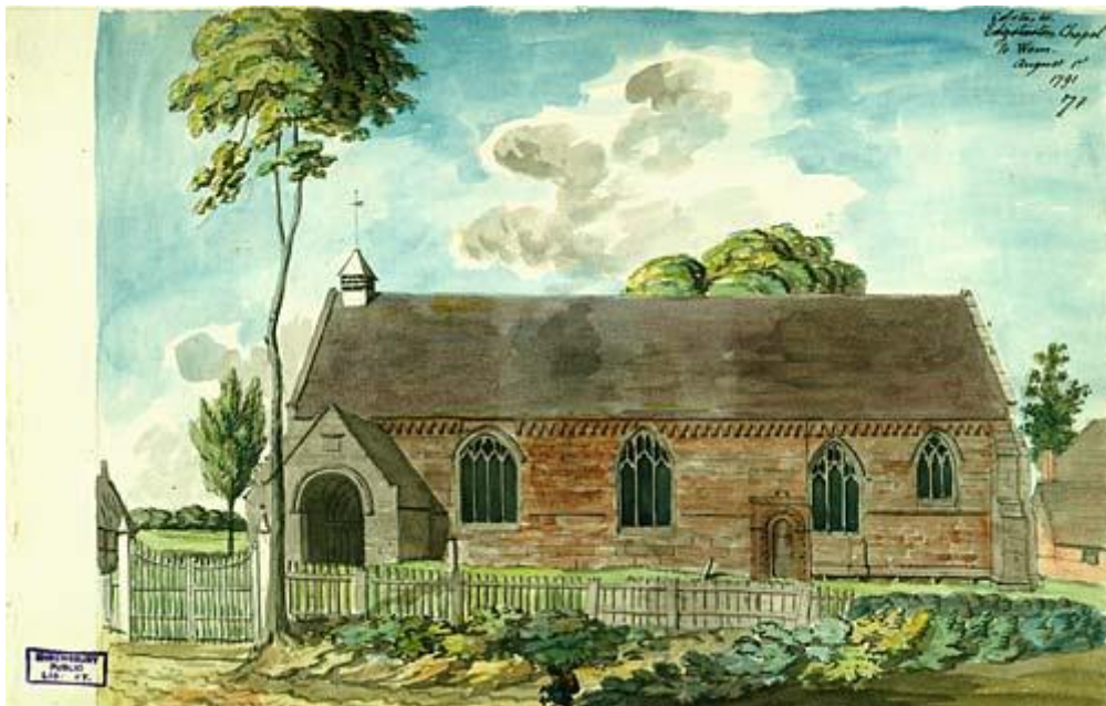
St Mary's Church, Edstaston before restoration in 1879
