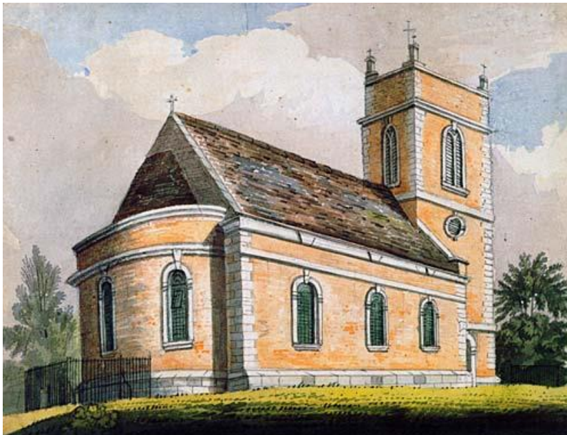
St Peter and St Paul church, Fitz before restoration in the 20 th century
