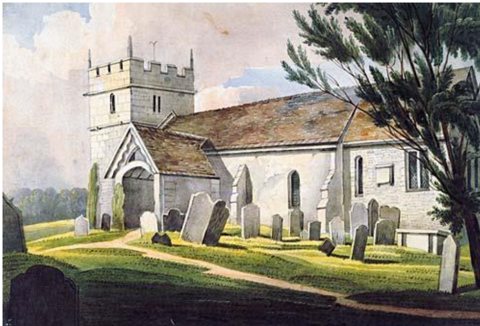
Church of The Holy Trinity, Holdgate 6009/104
